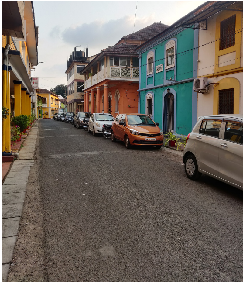
Figure 4: Local street in heritage area of Panaji
